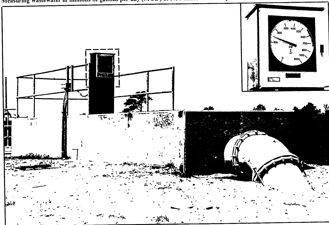
Measuring wastewater in millions of gallons per day (MGD) at New Hanover County's Southside Treatment Plant.
