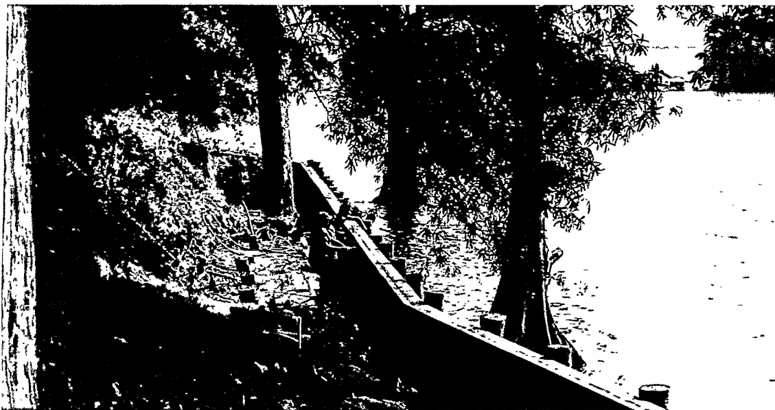
Bulkheads can be designed in ways that will preserve natural features, such as these cypress trees, and still effectively control erosion.
