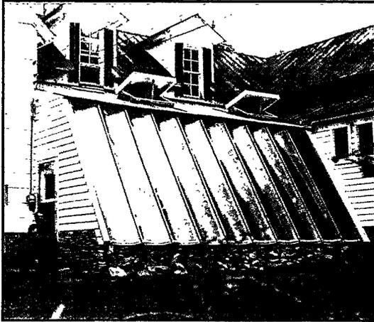
collectors, heat transfer fluids, or sophisticated electrical equipment — by passive systems. New homes are now being designed with large windows on southern exposures to bring in the winter sun and with carefully angled roof overhangs for summer shade. For existing homes — and for new designs — building a greenhouse on the south side of a house can achieve the same results.
